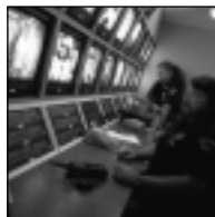
Video Surveillance (CCTV)
