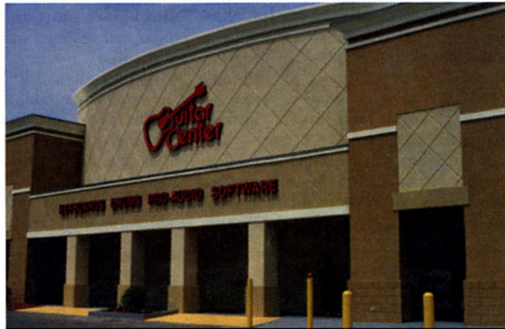
Forced side door and back door break-ins drove Guitar Center to install exit-only hardware to reduce shrink.
